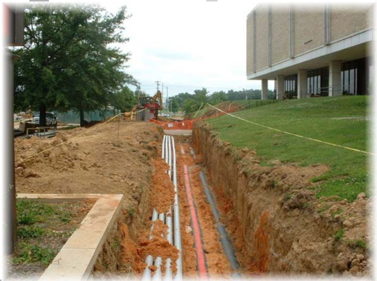
Construction of the campus district cooling east of Agriculture and Lab Science Complex.
